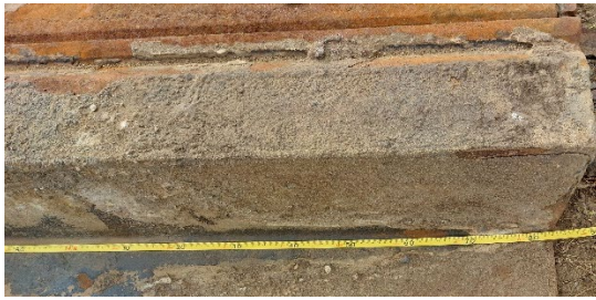
a) cleaning by the contractor with high pressure water jetting.
