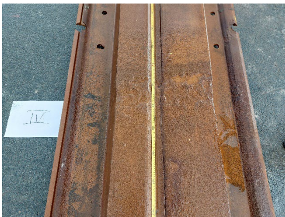
c) by Straalbedrijf Schep by means of sandblasting.
