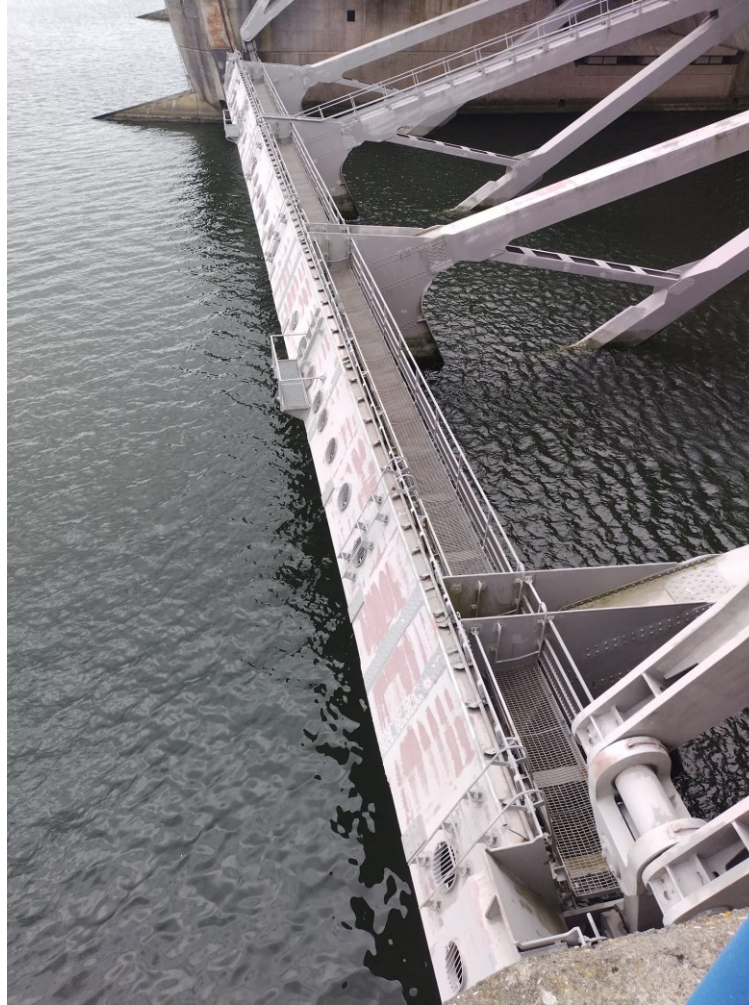
conservation layers of the segment sliders of the Haringvlietsluizen
