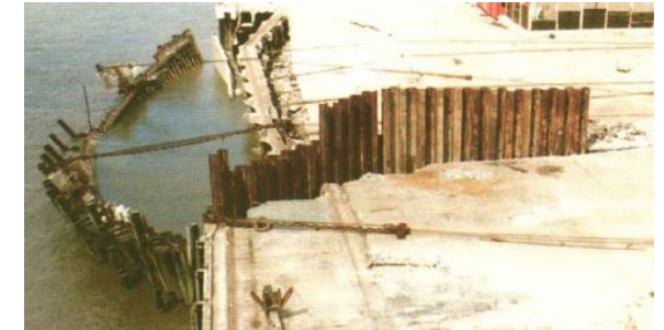
Pull-out failure of tendon/grout bond
