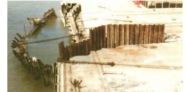
Pull-out failure of tendon/grout bond
