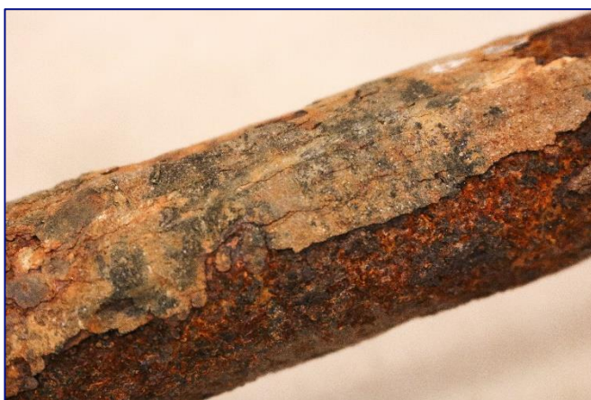
Figuur 77 Corrosie product detail anker Loofr-1.
